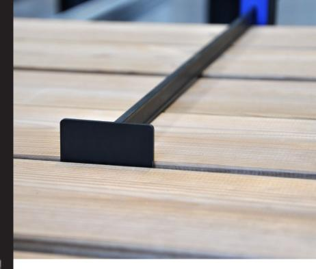
The **HELPO decking clamp** is a useful installation accessory for laying of decking boards.
